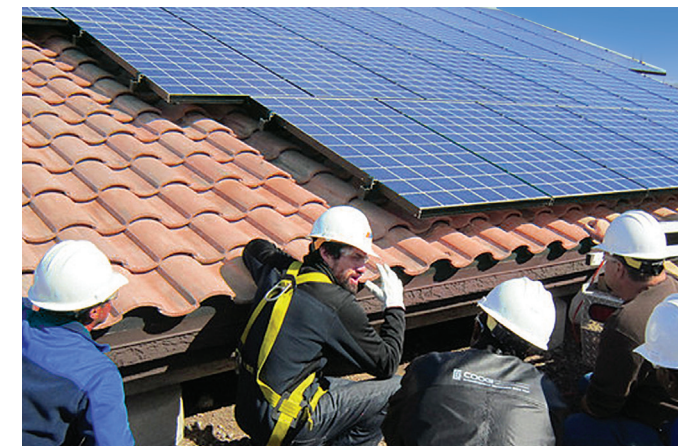
The company also provides on-site instruction for leading solar training organizations such as Solar Energy International.
